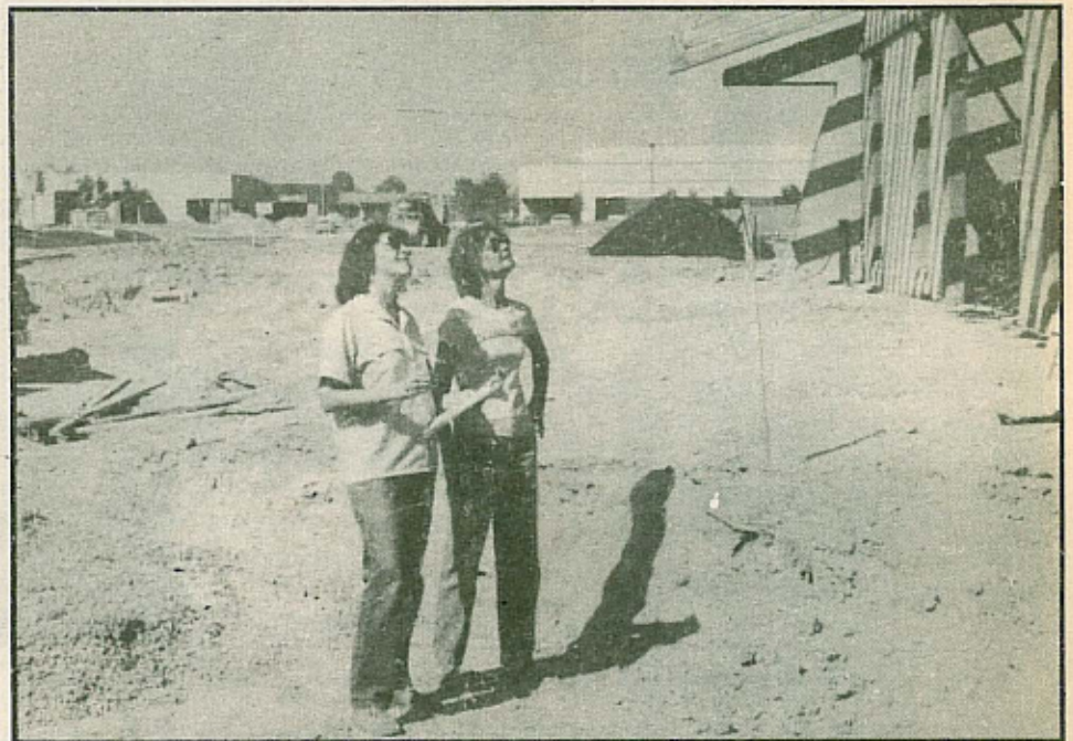
Inspectors Judy Myrick (left) and Betty McDaniel on the job at Valley Business Park.
